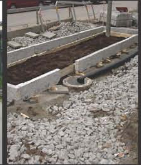
Large stones under paving
