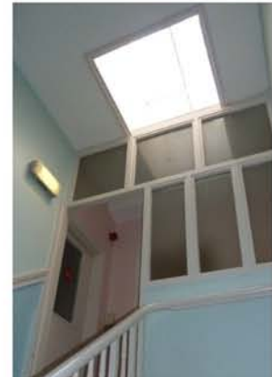
View of existing roof light
