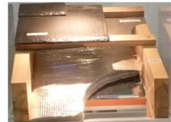
Retrofitting insulation under rafters
